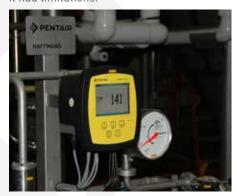
Haffmans' CCR allows Summit to supplement natural carbonation while processing. This saves time and preserves the desirable characteristics of the beer.
