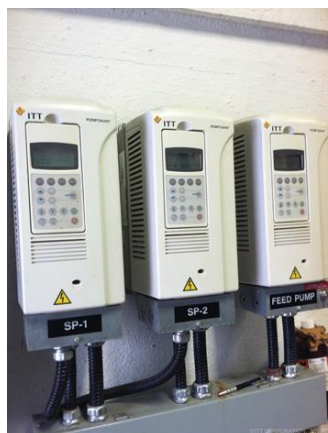
Figure 4. Units such as these control motor speed by changing the frequency supplied to the motor.
